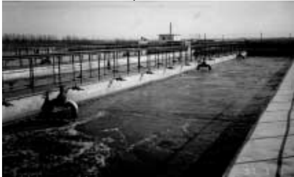
Figure 3 A/O aeration basin
