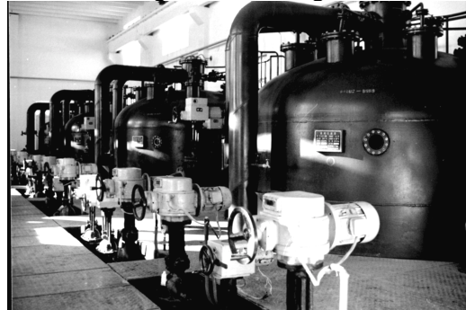
Figure 4 Pressurized fibrous filters for micro-flocculation contact filtration
