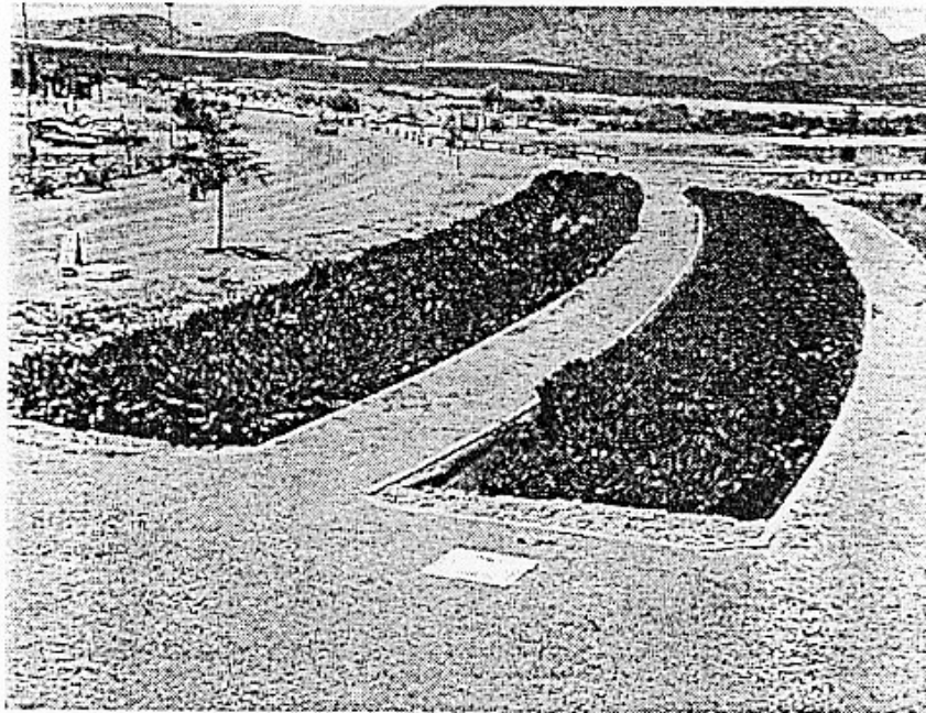
Canna lilies/Rock filter for sanitary secondary effluent advanced treatment.
