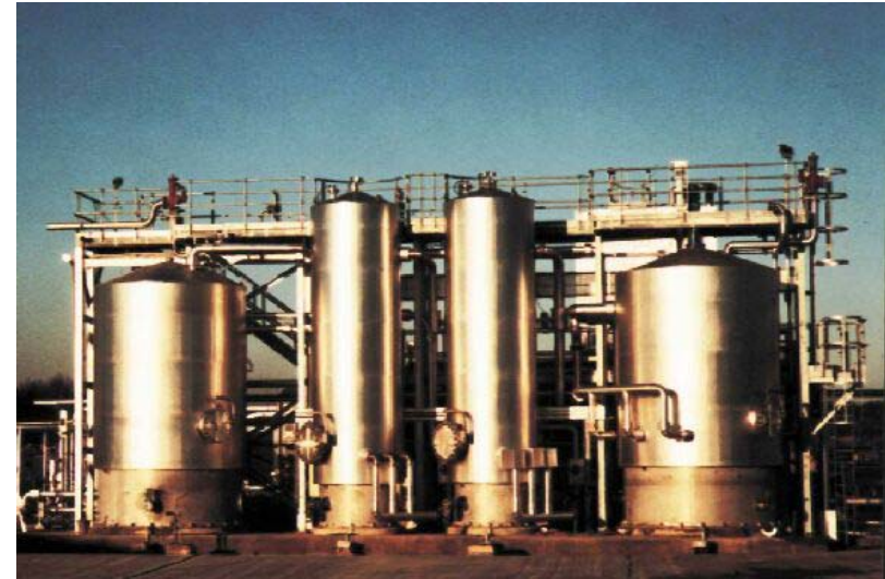
The CAMBI thermal hydrolysis process
