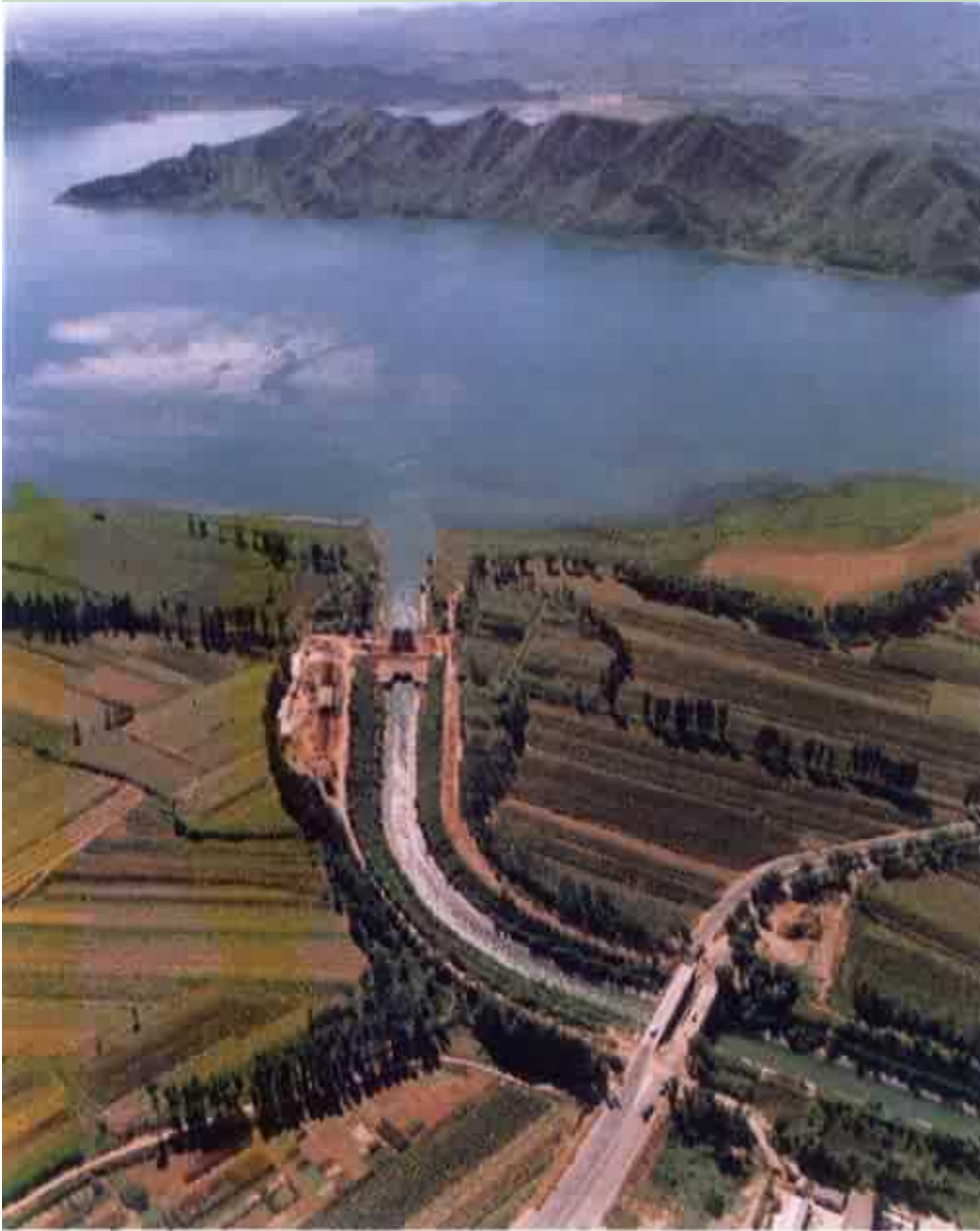
A Photo of transferring water from Huairou Reservoir to Beijing through Jingmi Canal
